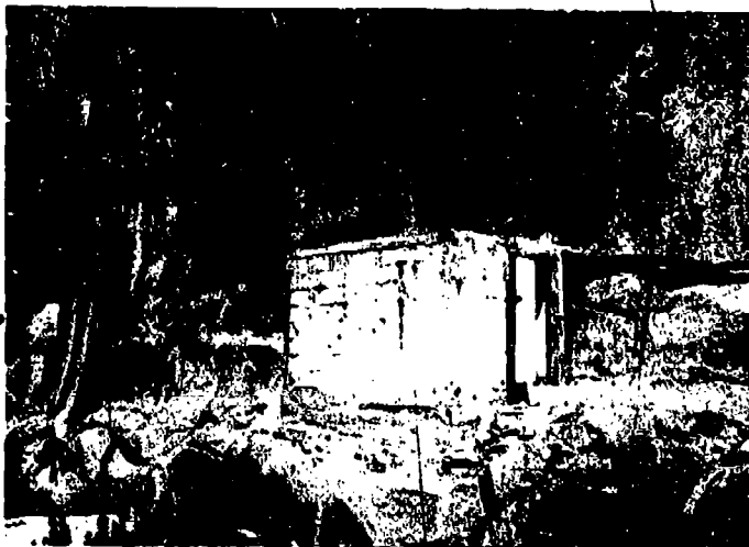
Vault containing recorders for seismic information in the Andes Mountains of northern Chile.
